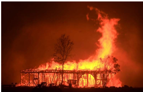
The Round Barn on fire. The firestorm encroached on all sides of the Keysite Campus but amazingly it was mostly undamaged.
