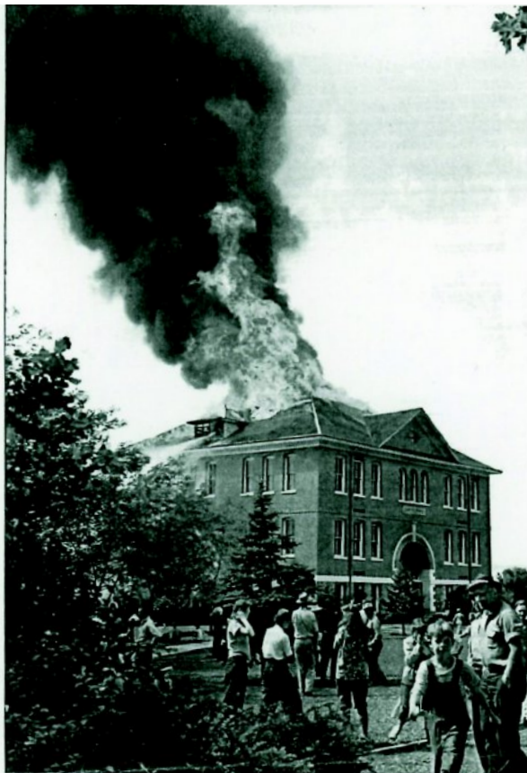
(Fire at Central School, 1947. Courtesy Compton Collection, USU Special Collections.)
