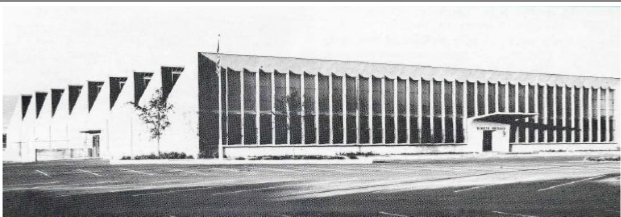
The corporate headquarters of the 1950 period was housed in Building 8, at the corner of Page Mill Rd and Park Blvd. Engineering and Sales was on the ground floor, Mahurin's Service Dept and Training group was in the basement. This was the first of the HP stylized "sawtooth roof" buildings, later used on the 6 buildings in Stanford Industrial Park on the hilltop in 1957.
