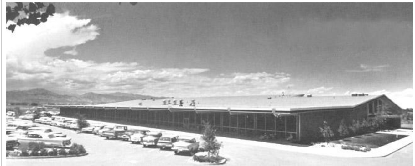
The HP Loveland Building in 1965 - From MEASURE Magazine, January 1965 - Courtesy of the Hewlett Packard Company
